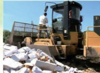
Disassemble packaging material waste transportation
